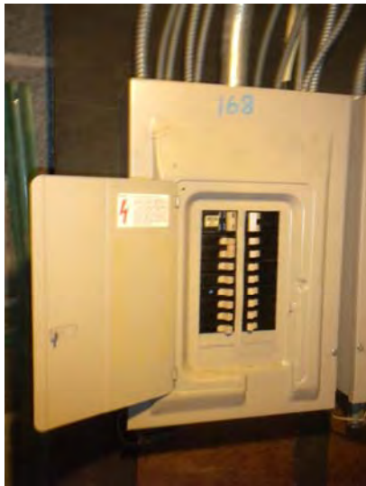
G/E circuit breaker panels are located in bulkhead rooms
