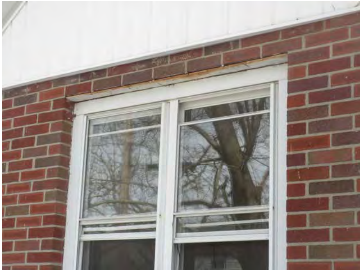
Rust noted on steel window lintels
