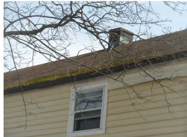
Isolated patches of organic growth were observed under overhanging tree limbs
