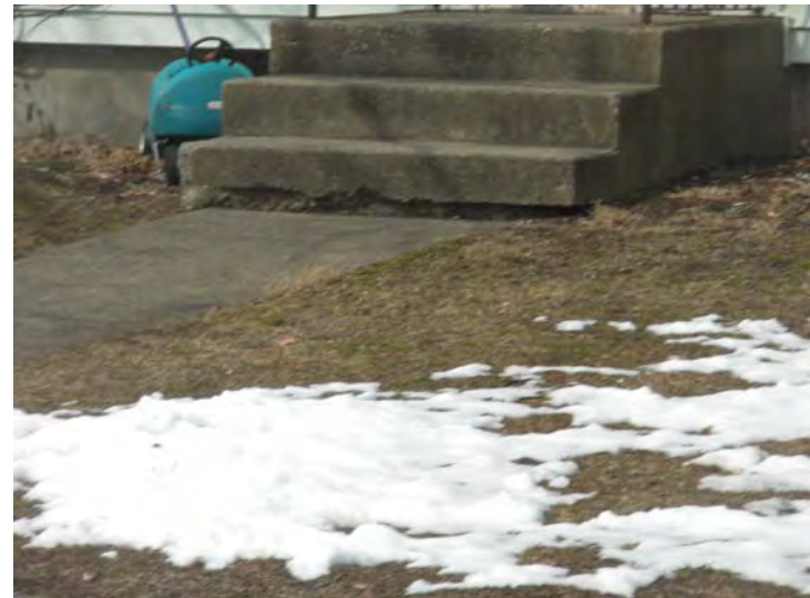
Typical deterioration of concrete steps at base
