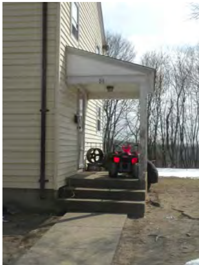
Some concrete steps are pulling away from the building. Note the leaning wood post.
