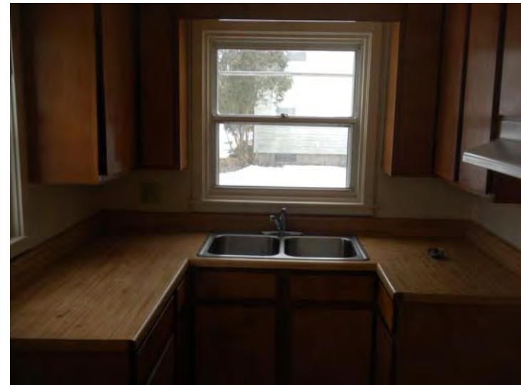
View of the original plywood cabinets with laminated particleboard countertops
