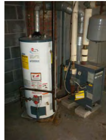
Typical domestic hot water and boiler configuration (located in basement)
